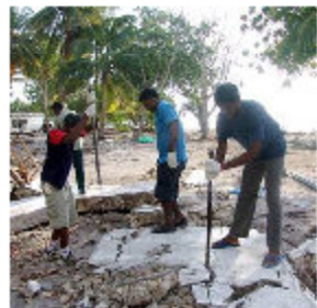
Damage caused by the 2004 tsunami Flickr_Tsunami Maldives
