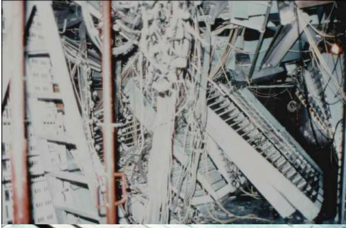
The top three floors of this communications building collapsed, cutting off domestic and international long-distance calls and significantly impacting local services in Mexico City after the 1985 earthquake.
